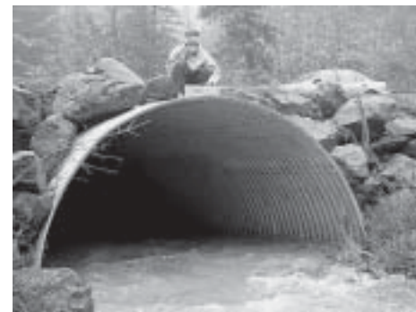
One of the many culverts surveyed on the Klickitat River.
